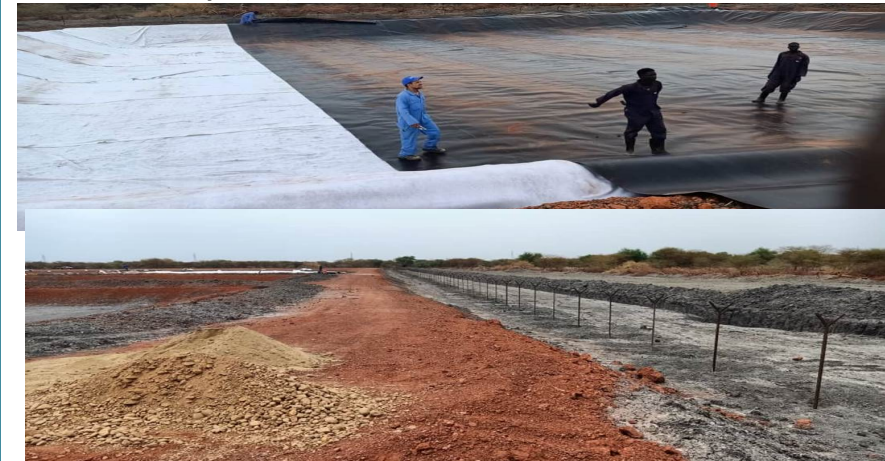
Project of Liner/Geo membrane Installation for contaminated soil treatment site ongoing with liner installation, fencing, gate installation May 2021)
