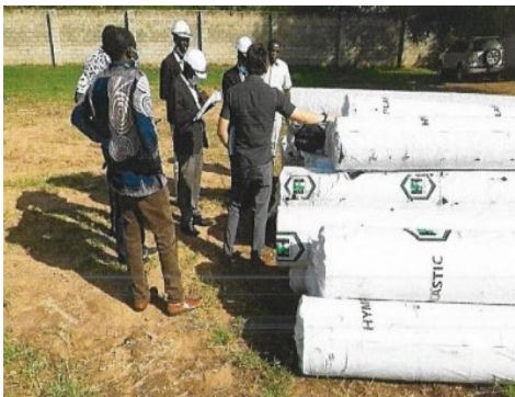
Material (liner) inspection for Unity contaminated soil treatment site (November 2020)
